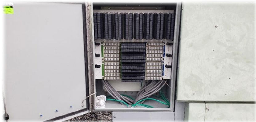
192 Port MAQS System with 96 Port Modular Cross Connect (P/N SA-7100-0201)
