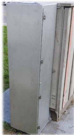
MAQS CuB 3 192-PORT Enclosure (P/N SA-7100-1501)
